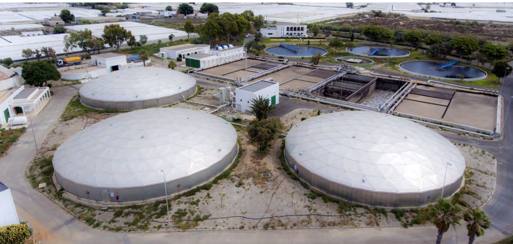
El Bobar Wastewater Treatment Plant (WWTP) in Almería (Spain).
