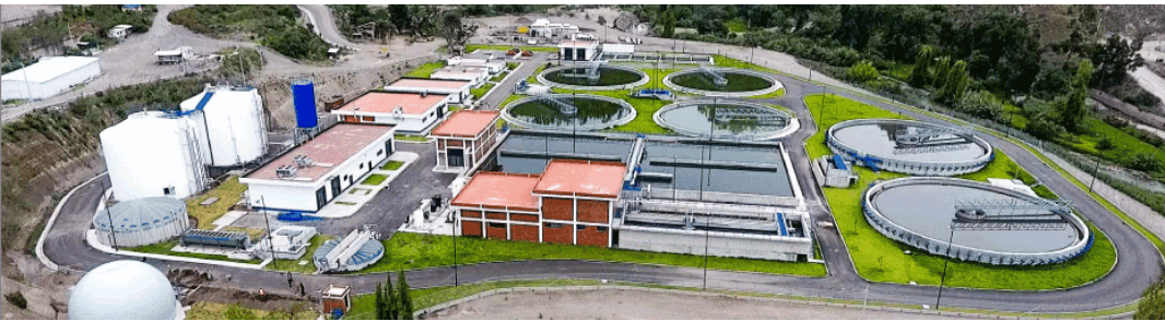
The AMBATO WWTP (Ecuador).
