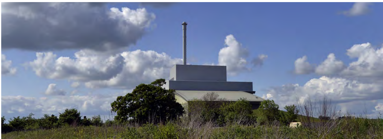
The Greatmoor Energy from Waste Plant in North Buckinghamshire, UK, serves over 40,000 local households.
